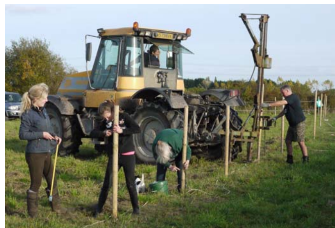
Reach Riders Arena under construction
