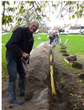
Electricity was installed on the Green
